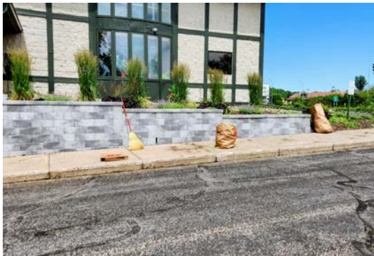
CWS Clean Up
